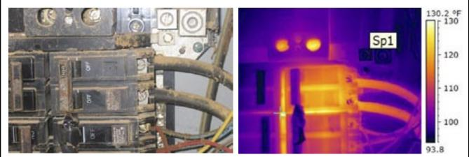
Photo set #3. Photo on left shows a 15 year old 150-amp power panel in a poultry house. The infrared photo at right shows the breaker is heated to about 130 degrees F, which means it is likely to fail or trip prematurely. The reason is that this breaker is feeding a second poultry house! Power should never be fed through one poultry house to another, but only from the farm main service.
