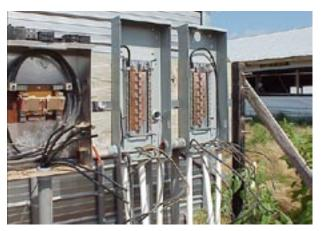
What's wrong with this picture? New electrical service and panels are being installed to handle the increased electrical load of an upgraded environmental control system – but the old wires leading from the panels are not being replaced. They will be undersized and likely to fail.
